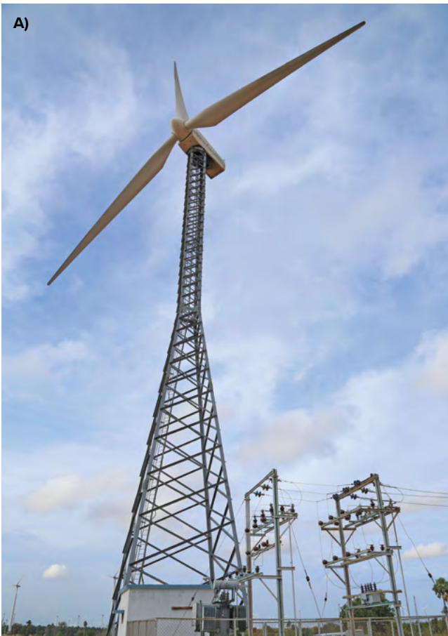
1.5 MW Wind Farm at Dharapuram, Tamil Nadu
