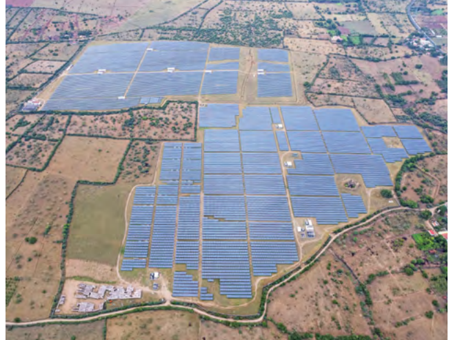
10 MW EPC projects at Erode District, Tamil Nadu
