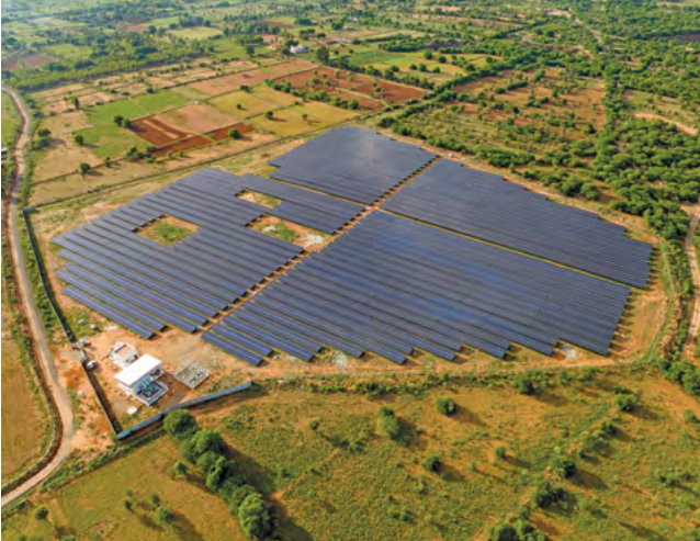
10 MW Solar Power Plant-Foundary at Dindigul, Tamil Nadu
