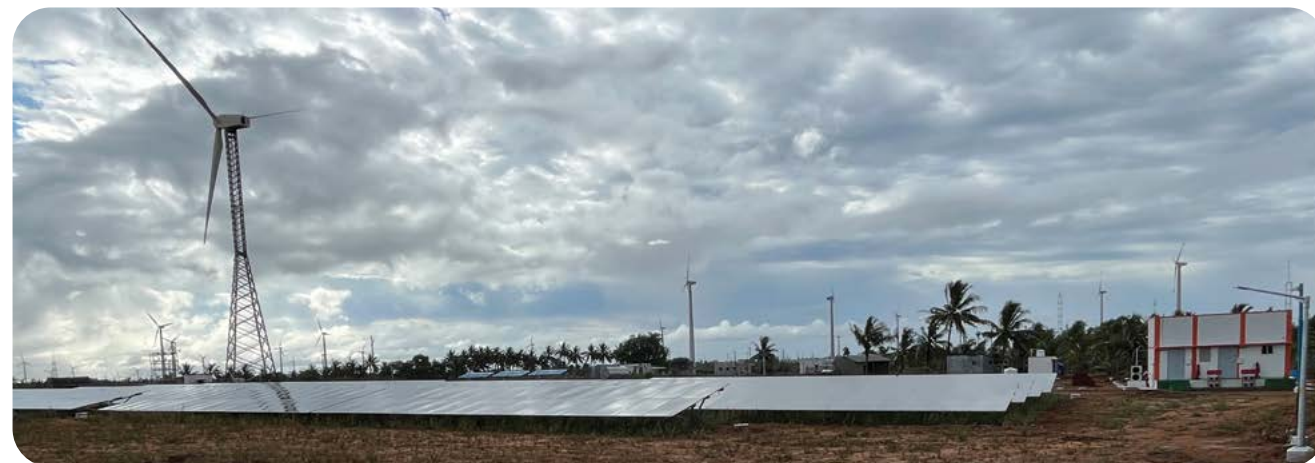
500 kW Wind Solar Hybrid with BESS Plant in Tirupur District, Tamil Nadu
